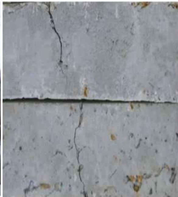
Fig: 4.6 Flexural crack
